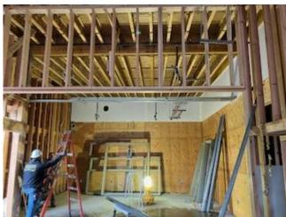
Interior framing nearly complete. Plumbing and electrical rough-in underway.
