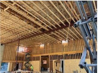
October 15<sup>th</sup>- The station is dried-in with vapor water barrier.
