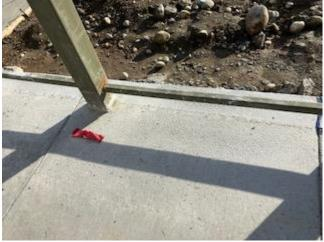
This pitted concrete has been rejected and will be replaced.
