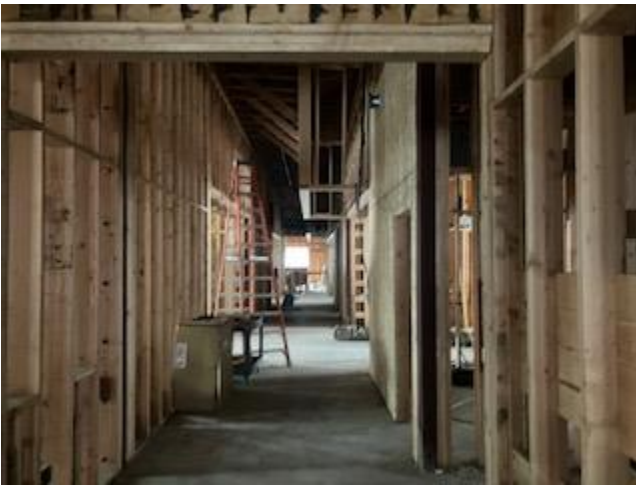
Interior administrative area framed out and drying out.
