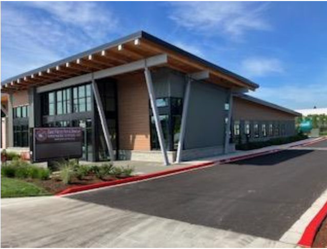
Pretty much complete, working through final permit approvals.
