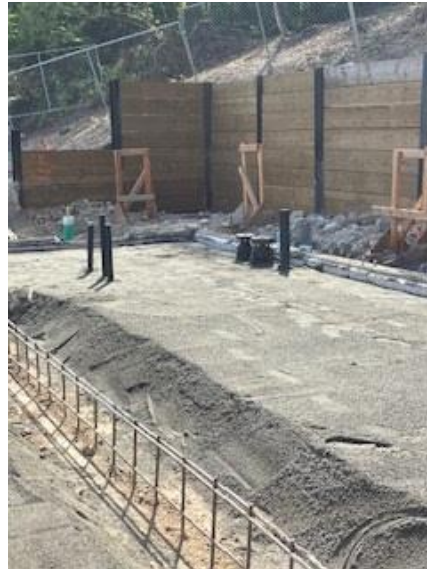
App bay and support area slab preparation
