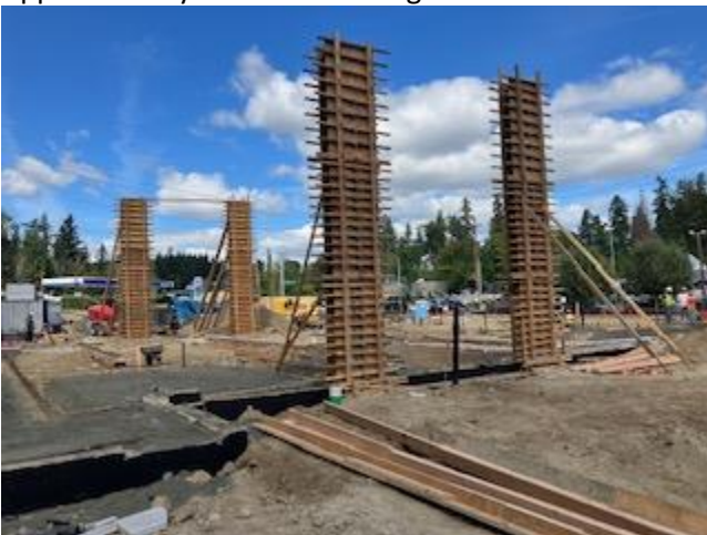
Apparatus bay columns forming.
