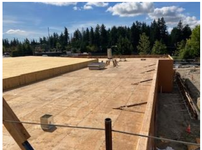
Admin area is topped out.
