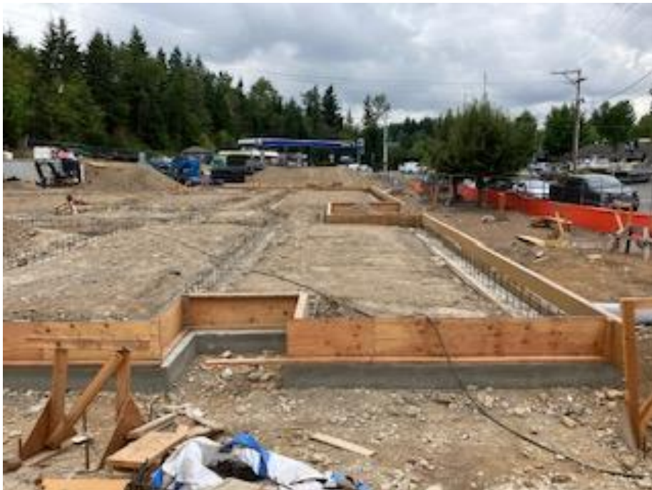
Foundation forming in the living quarters.
