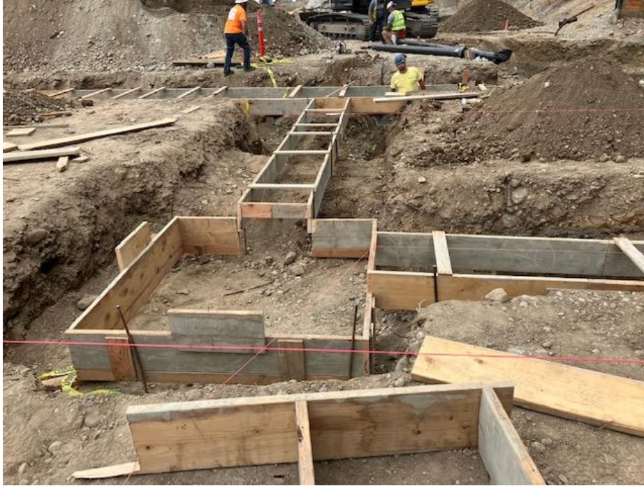
Footings and forms in the apparatus bays.
