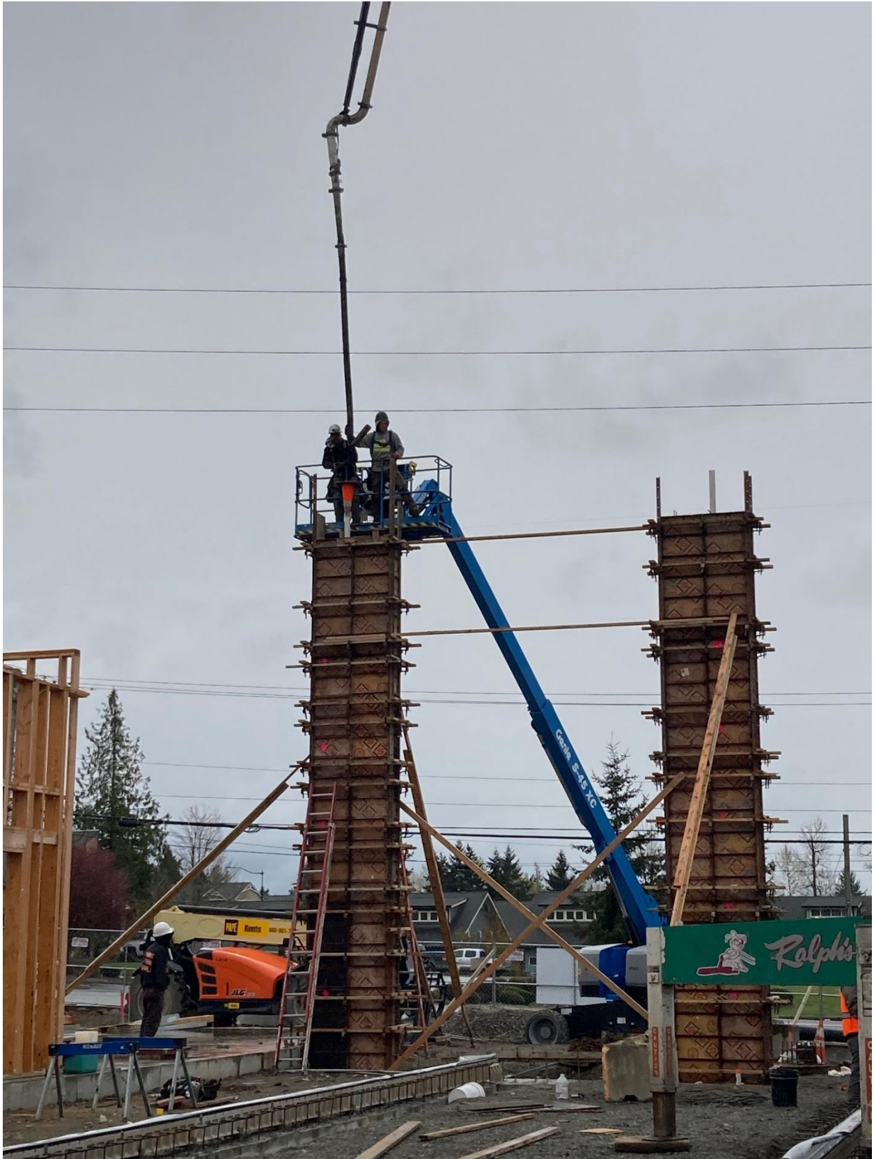
Pouring the 20-foot-tall pillars that frame the apparatus bay doors
