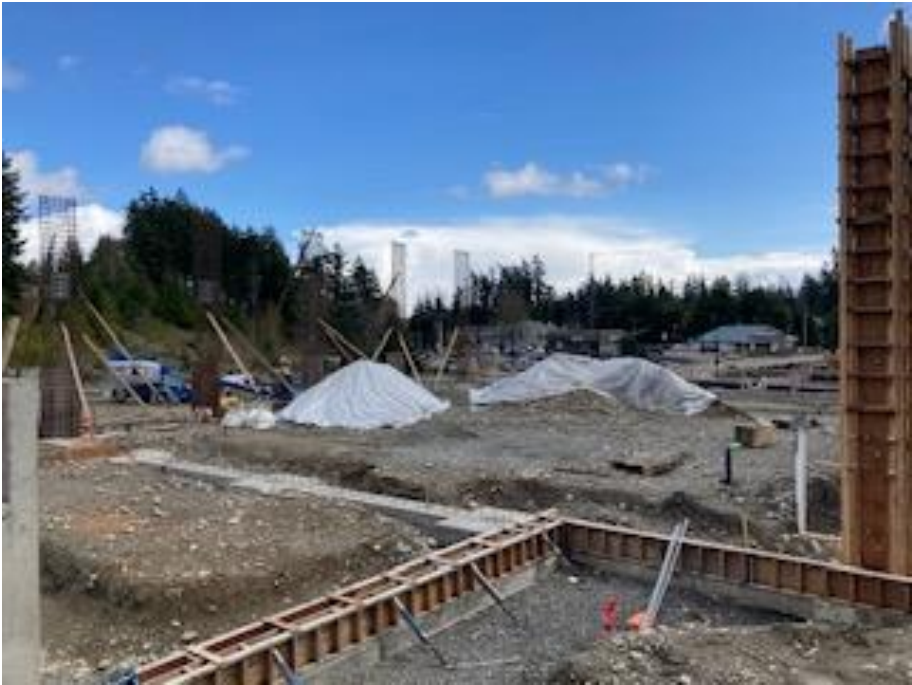
Rebar for the north apparatus bay columns.
