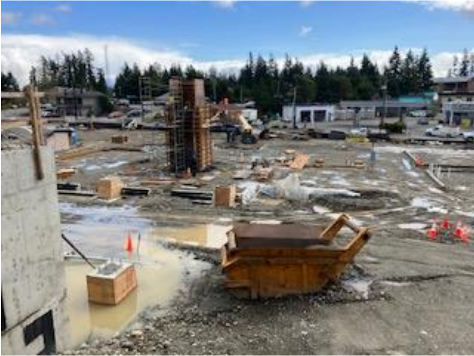
2 nd floor of the elevator shaft being formed.
