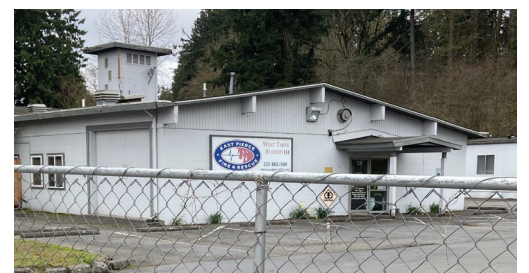
Lake Tapps Station 114 is vacated and under construction.
