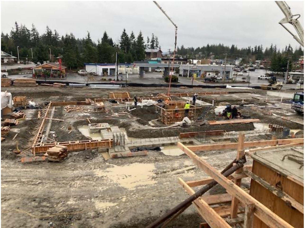
First of the admin foundation walls
